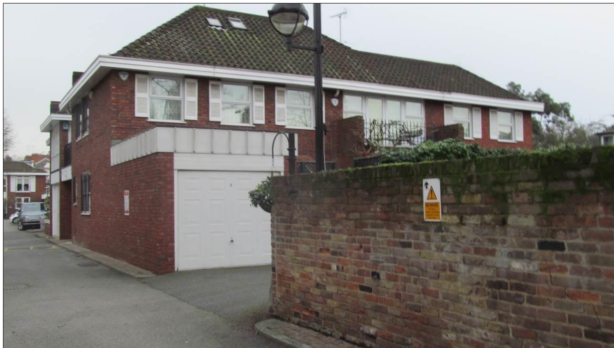
Front elevation of No 14
