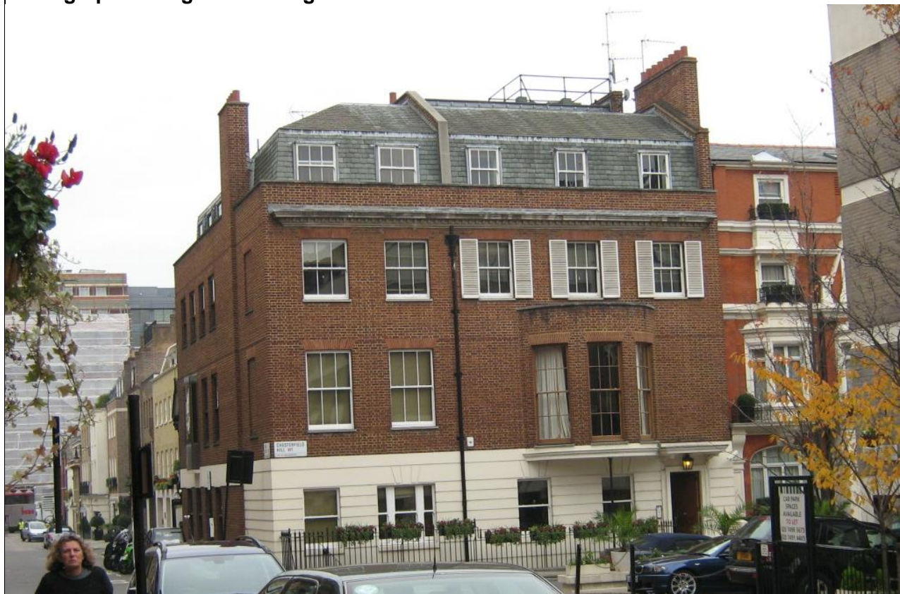
Photograph 1: Original building before demolition
